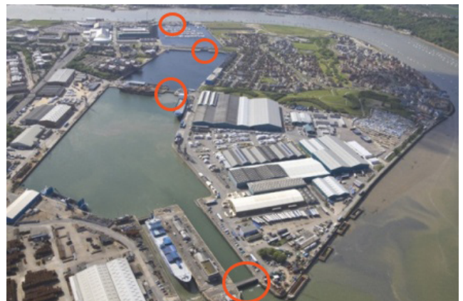
Location of the four watertight lock gates at the Chatham Historic Dockyard. Photograph courtesy of Peel Ports.
